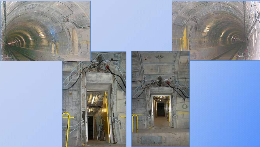
Completed cross-passage construction
